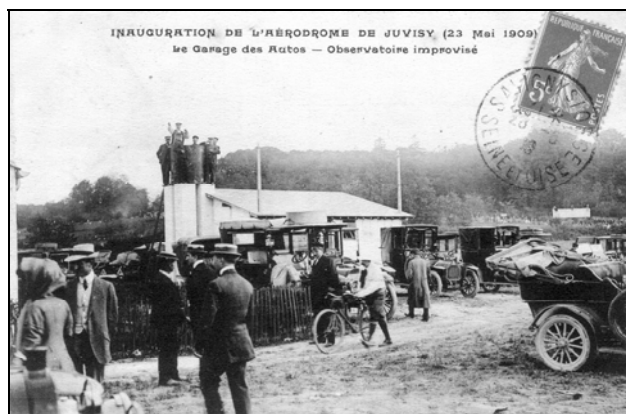
An improvised observation post in the parking area
